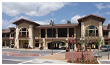
Building 3 Central View
