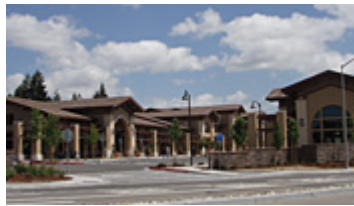
Bldg 3 & 4 South Corridor
