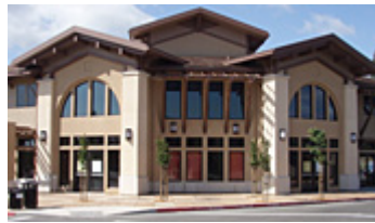
Bldg 1 Front Entry
